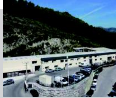
RAGNI headquarters in Cagnes sur mer, France
