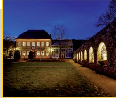
Staged to perfection with luminaires and LED modules by Arne Fiedler and VS.
